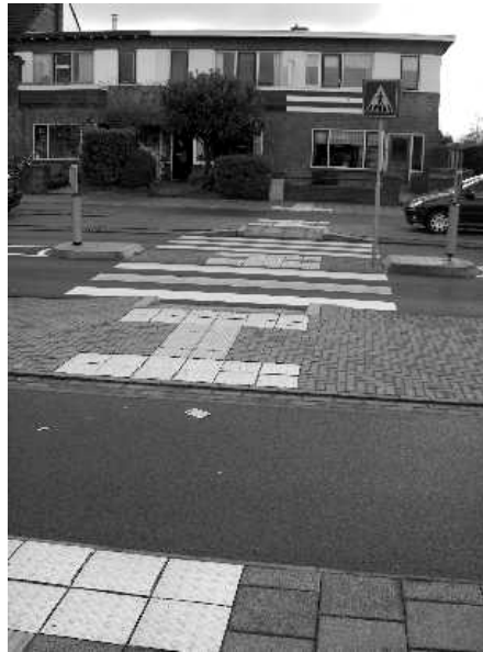
Guided lines for the visually impaired
